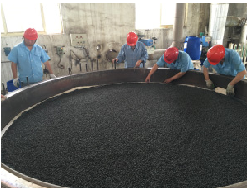
Installation of Clariant's secondary N 2 O abatement catalyst EnviCat® N2O-S in a medium-pressure nitric acid plant.
